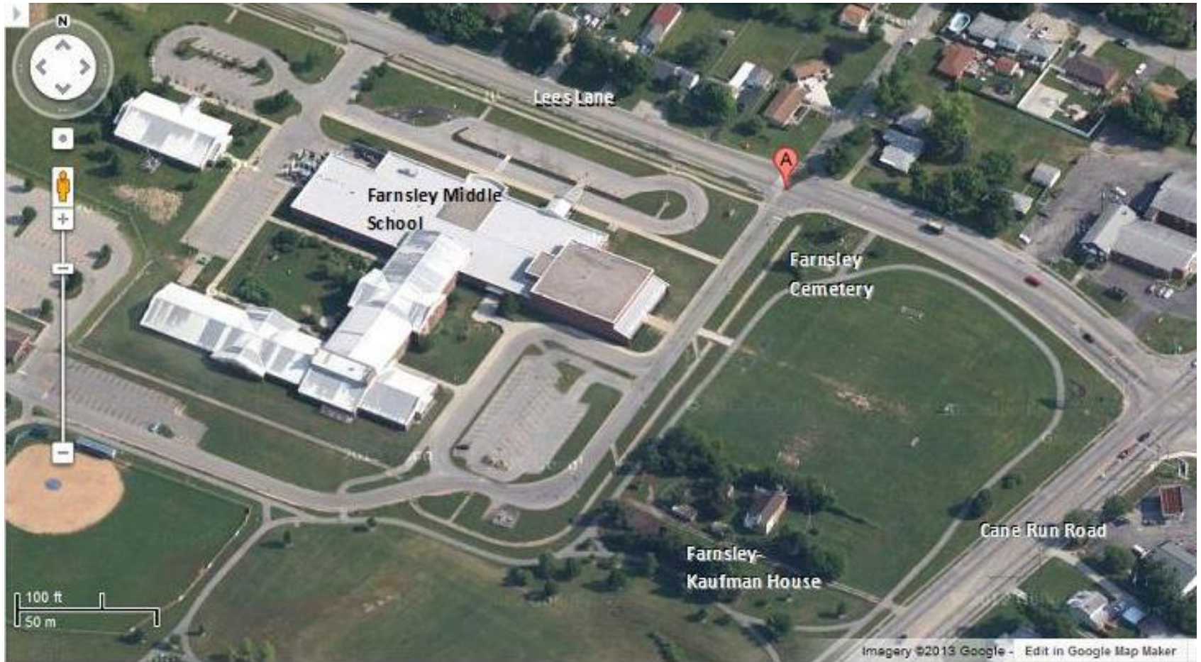
Figure 1. 2013 Google aerial showing the location of the Farnsley Cemetery.
